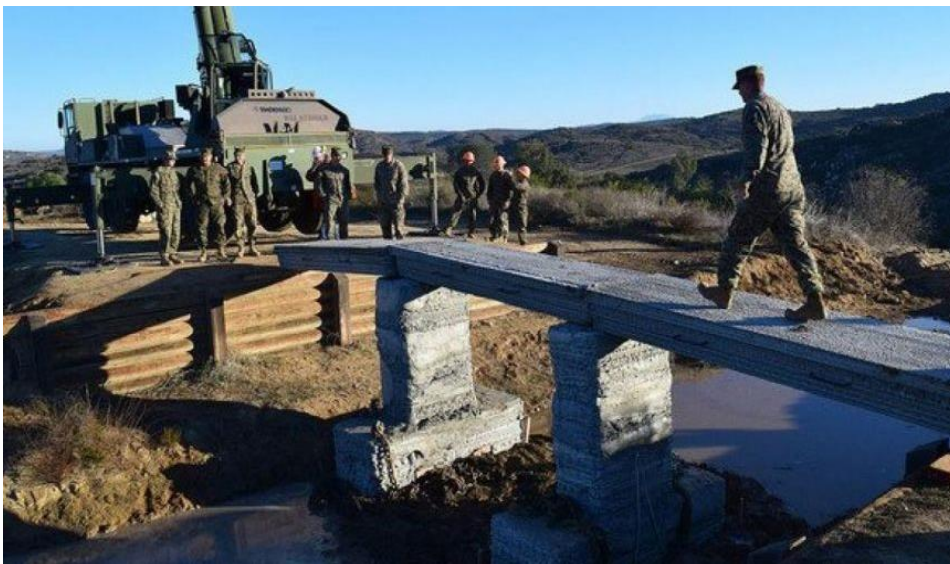
Figure 2: 3D Printed Concrete Bridge.
