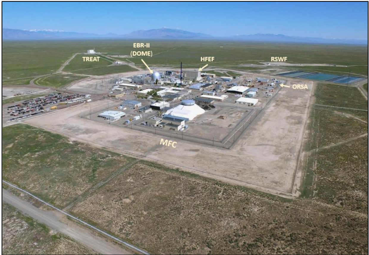
10 11 Key: DOME = Demonstration of Operational Microreactor Experiments (formerly known as the EBR-II [Experimental Breeder 12 Reactor II] test bed); HFEF = Hot Fuel Examination Facility; MFC = Materials and Fuels Complex; ORSA = Outdoor Radioactive 13 Storage Area; RSWF = Radioactive Scrap Waste Facility; TREAT = Transient Reactor Test Facility
